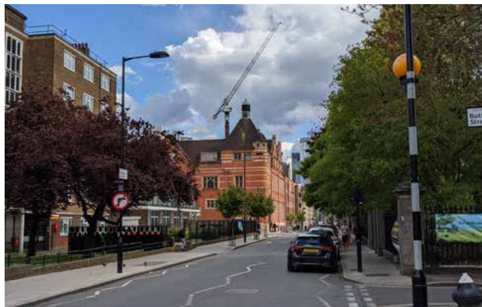
40 Pitfield Street (Former Library) funded by John Passmore Edwards (Grade II Listed)
